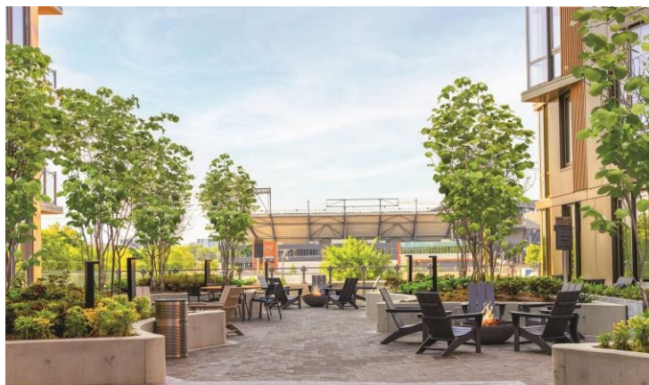
River Point | LEED Gold | Photo: Ray Cavacchio
