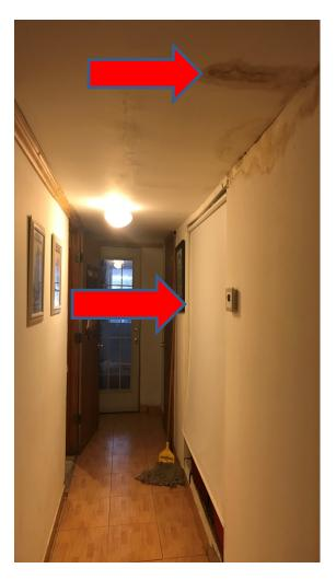
Moldy drywall by bathroom, kitchen, and hallway. Additionally, the Combustion Appliance Zone (CAZ) was not properly closed off.
