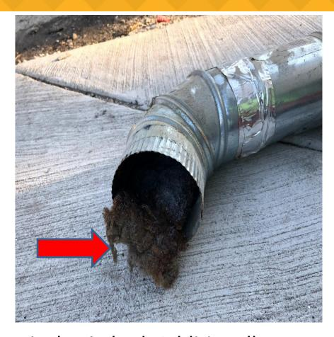
Domestic Water Heater is negatively pitched. Additionally, we found the flue pipe had material blocking the full use of the pipe.
