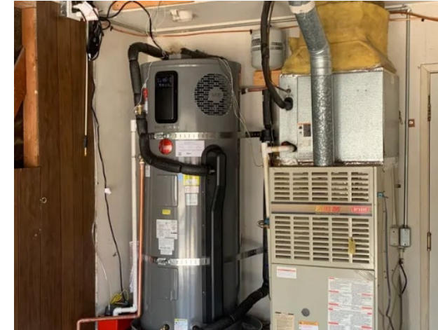
120V heat pump water heater field study cosponsored by Focus on Energy & Consumers Energy
