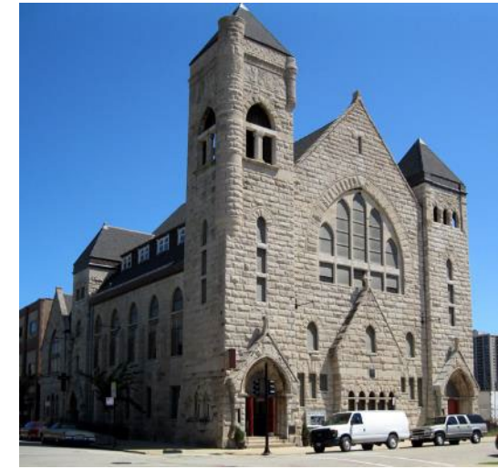
VRF heat pump demonstration completed at historic Quinn Chapel AME church
